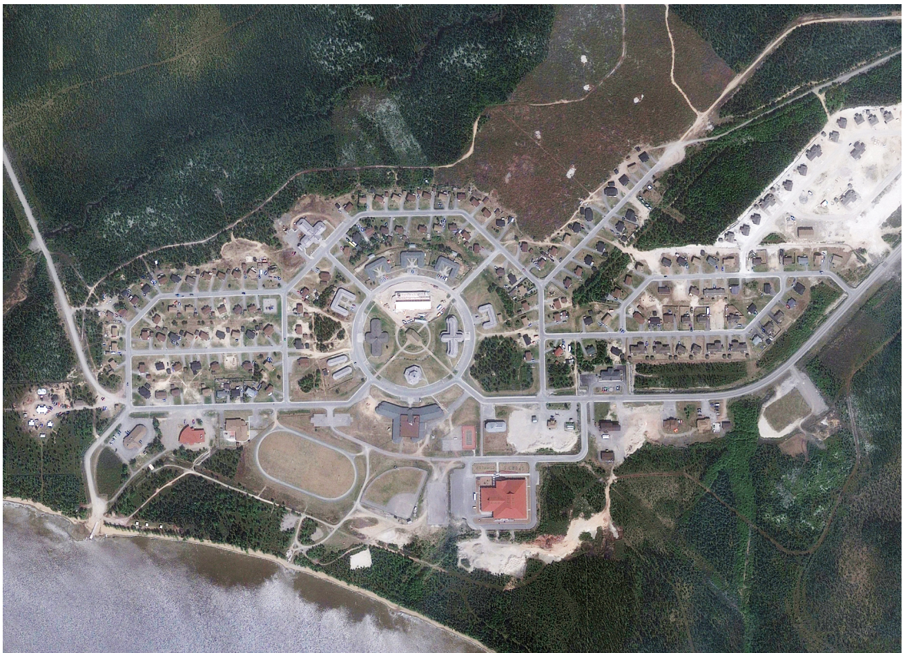
Figure 3. Oujé-Bougoumou, Quebec. Radial grid formed in the development of the new Oujé-Bougoumou community. Source: Author with base from Google Earth.
