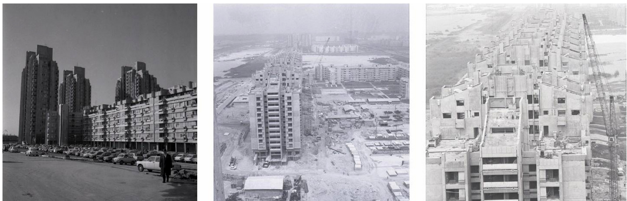
Figure 1. Photo-collage of Block 23. Note: The first image shows the completed Block, while the following two display it during construction with a focus on building no. 6. Source: “Fotografije blokova 22 i 23” (1975).
