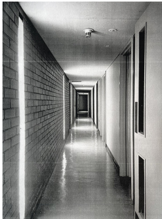
Figure 6. Internal corridors. Photo courtesy of Ryder Architecture.
