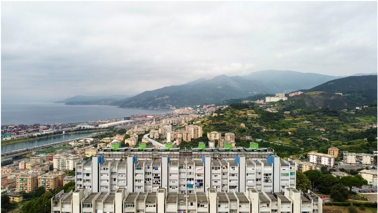
Figure 3. Le Lavatrici housing complex (The Washing Machines) and the Prà district, 2022.
