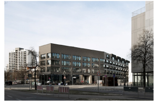
Picture 2. Integrated building project at the former Blumen-großmarkt (iBeb). Source: Andrew Alberts, Heide von Beckerath, 2016.
