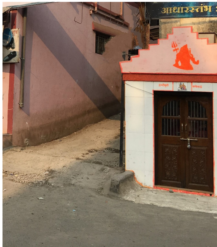
Figure 4. A mandal constructed at a crossroad.
