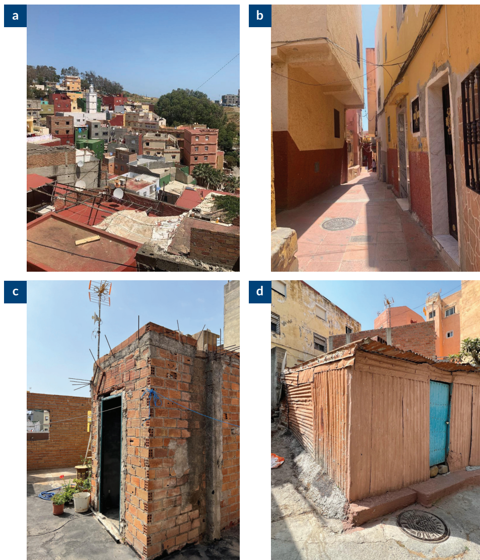
Figure 3. Constructive tactics at El Principe. (a) El Principe's eastern sight depicts its under-construction character and alley, (b) revealing the horizontal expansion thanks to cantilever beams; (c) exposed rebar; and (d) the corrugated metal sheets concealing the construction process. Photos by the author.
