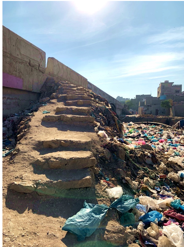
Figure 5. Stairs leading to Lyari Expressway.
