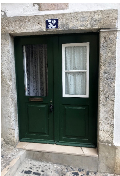
Figure 1. Door wicket and threshold, Alfama, January 2020.
