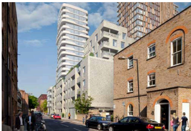
Figure 8. The Whitechapel Estate proposal permitted by the Secretary of State in 2017. Source: PLP Architecture and Adjaye Associates in Dunton (2016).
