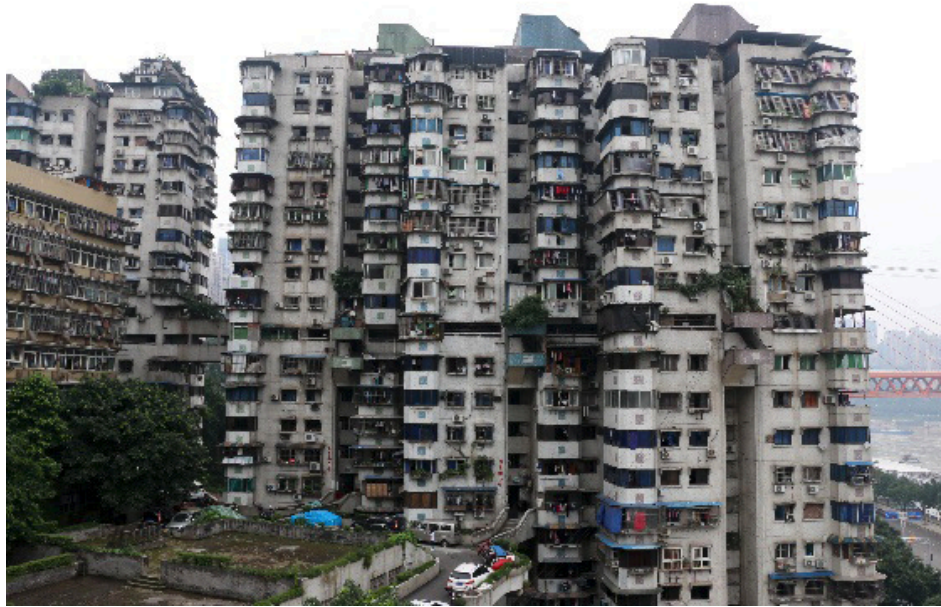
Figure 4. Baixiangju residential complex.
