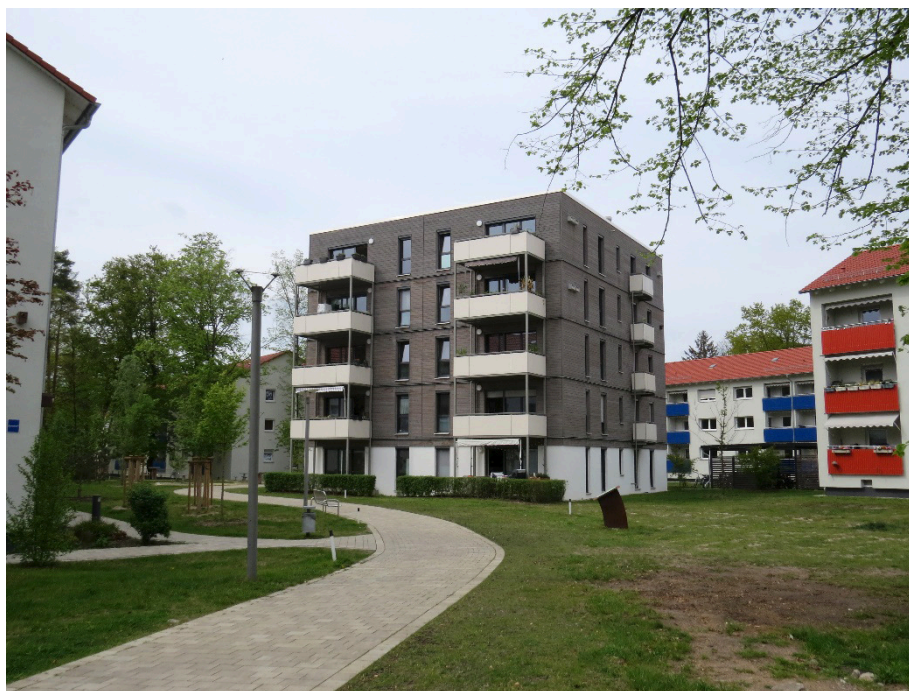
Figure 4. Newly arranged area of the Rathenausiedlung, now renamed Jaminpark.
