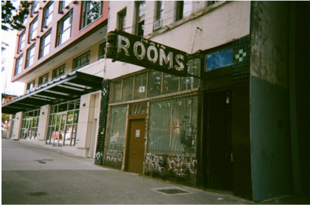
Figure 4. SRO housing. Source: Photo credits, Juan.
