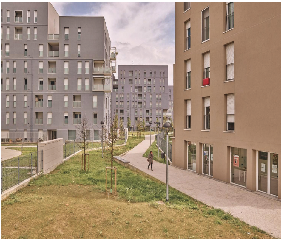
Figure 6. The ground floor spaces of WeMi Voltri (on the right) inside the social housing estate of Via Voltri-Via di Rudini, Milan. Source: Courtesy of Giovanni Hänninen.
