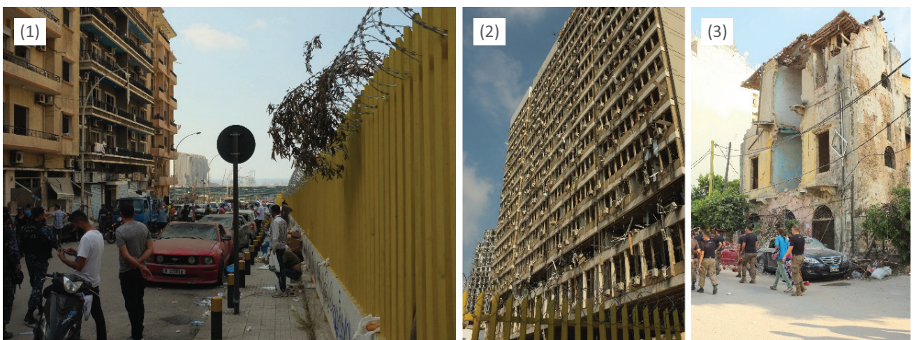
Figure 10. Photographs of the area after the blast: (1) Observing the silo from a distance, (2) Electricité du Liban, and (3) destroyed colonial houses.
