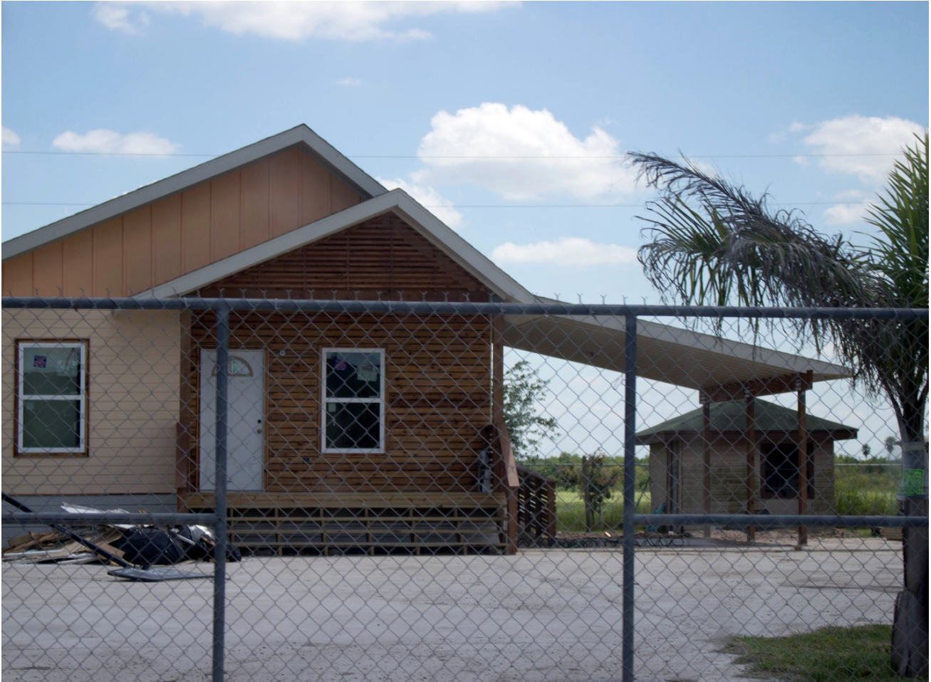
Figure 3. Nearly completed RAPIDO prototype home, designed using a sustainABLEhouse model, under construction in a colonia north of Weslaco, Texas. Source: Author (2015).
