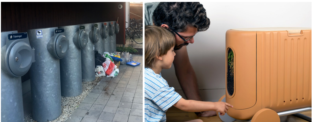
Figure 1a. A vacuum system for waste management in Kvillebäcken, Gothenburg. Photo credits: Pernilla Hagbert. 1b. Super Local Heating. Photo credits: David Molander.
