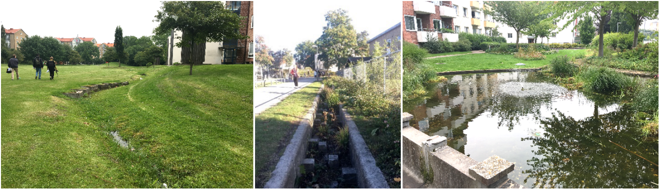
Figure 2. From left to right: Sunken lawn (part of Augustenborg remodelled park); one of the paved canals; one of the wet ponds. Source: Misagh Mottaghi.
