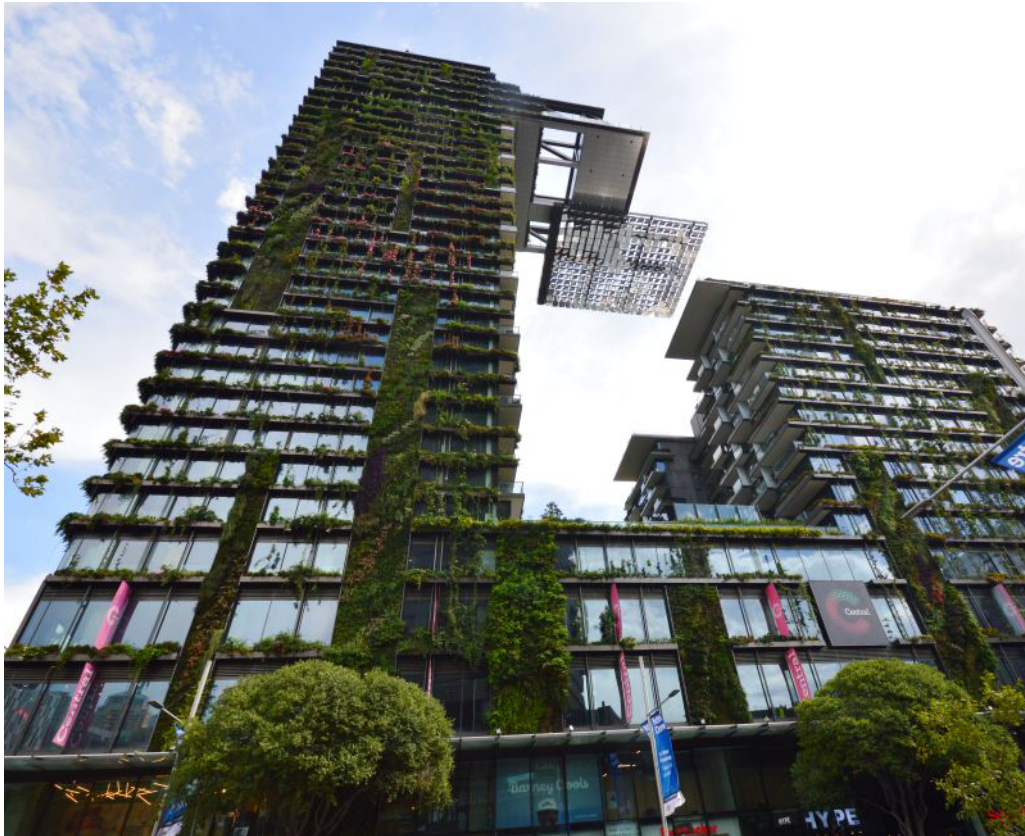
Figure 6. Central Park One. Source: www.frasersproperty.com.au
