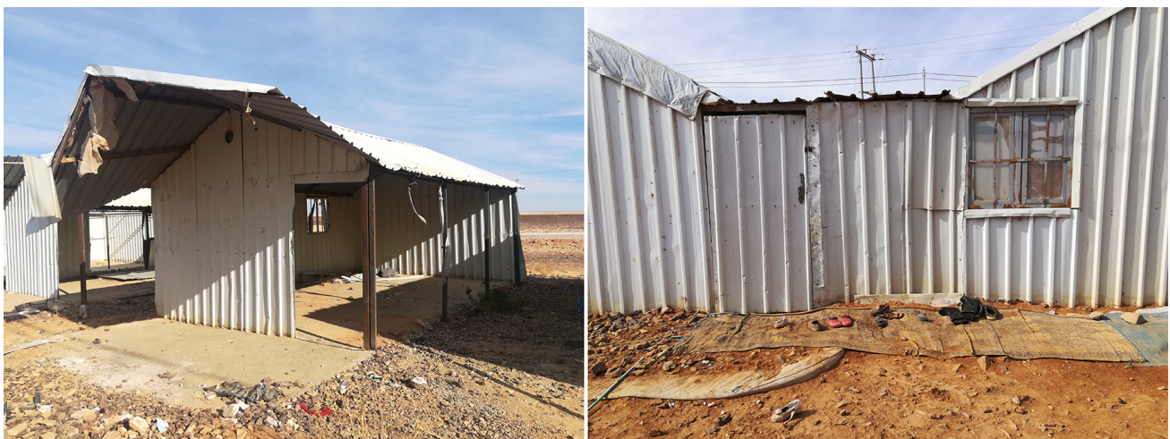
Figure 4. The vandalism of uninhabited shelter units to appropriate inhabited ones and connect them to create additional spaces. Source: Dalal taken in 2018.
