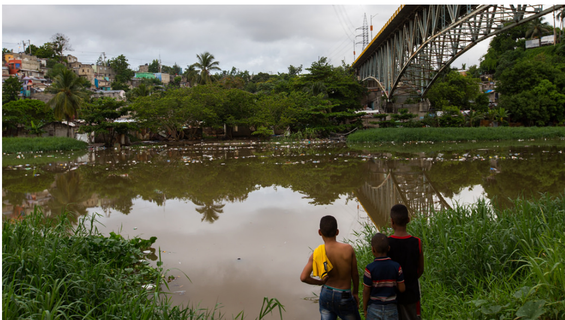
Figure 3. La Vieja Barquita neighbourhood and the Ozama River in Santo Domingo. Source: URBE (2017).
