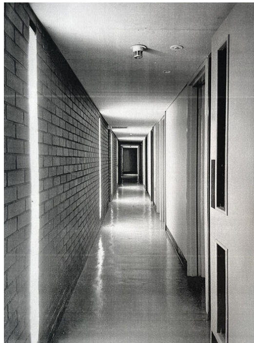
Figure 6. Internal corridors. Photo courtesy of Ryder Architecture.
