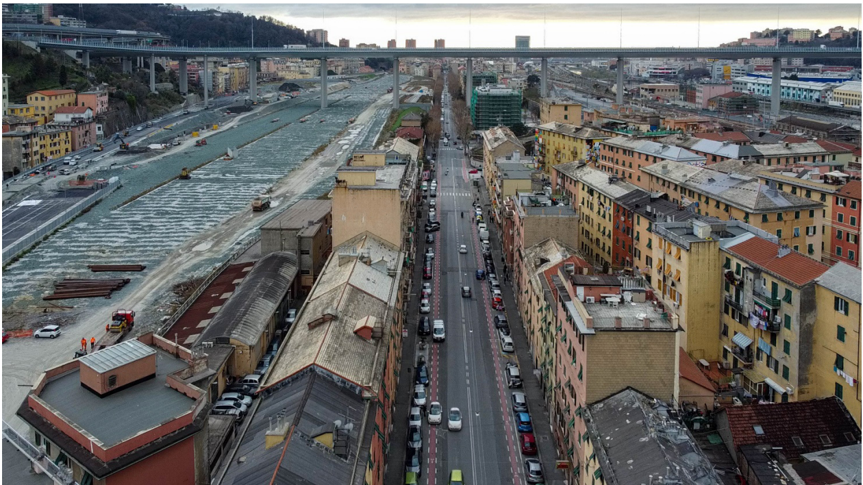
Figure 7. The new San Gregorio Bridge and the Sampierdarena and Certosa districts, 2023.
