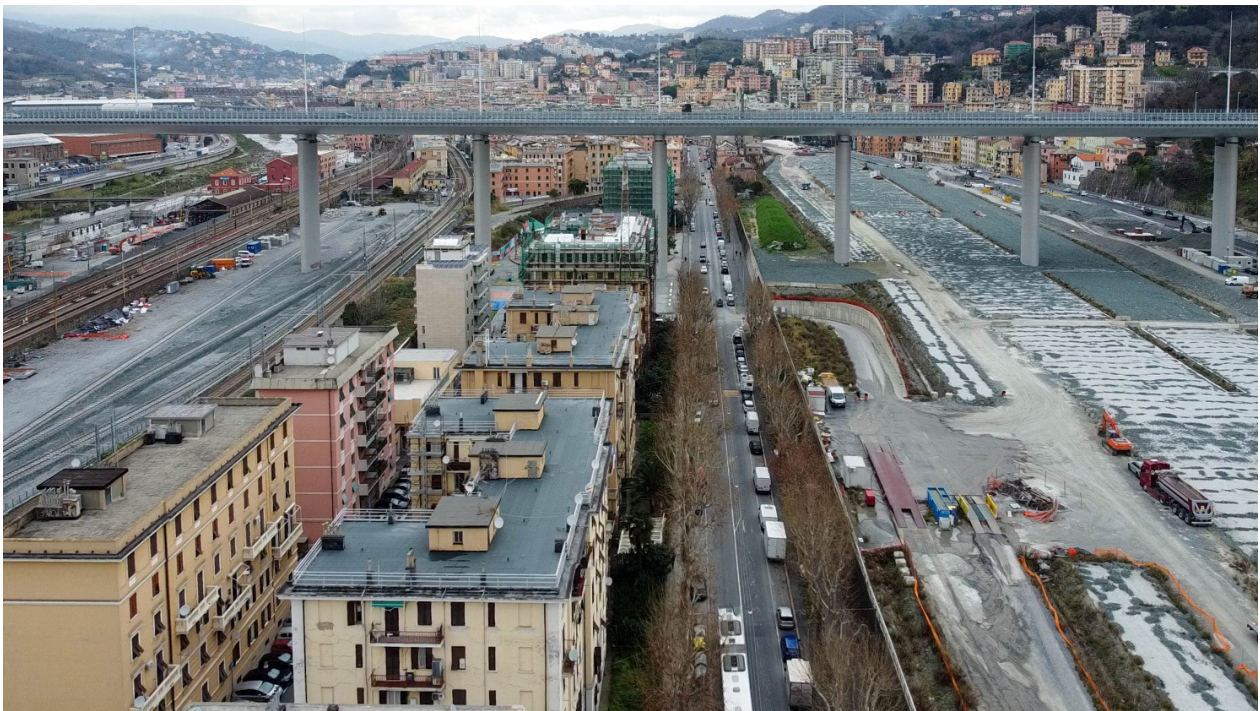
Figure 6. The new San Gregorio Bridge and the Sampierdarena and Certosa districts, 2023.
