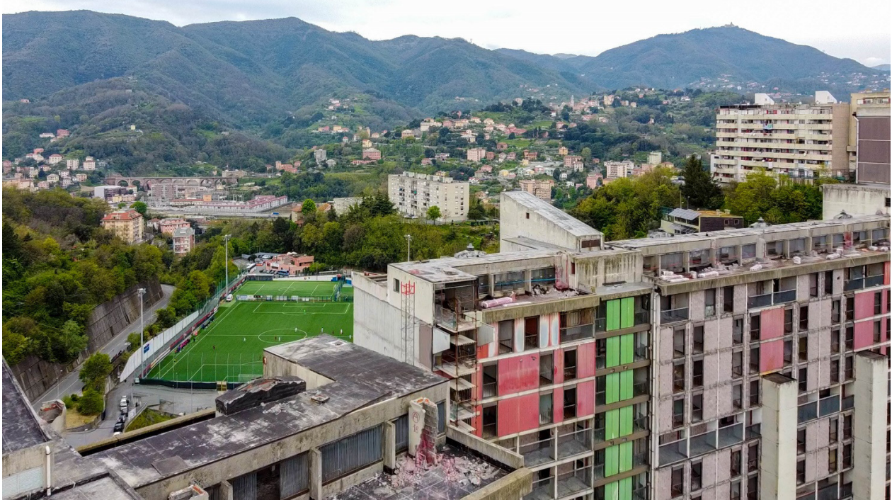
Figure 4. Diamante district, Valpolcevera, and Begato Dam during dismantling and demolition, 2021.
