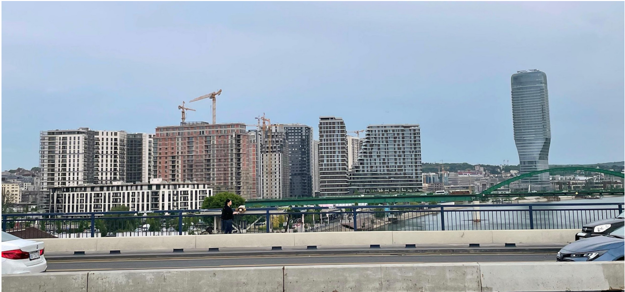
Figure 2. View over the BW construction site.
