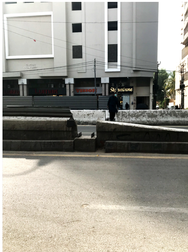
Figure 4. Walking pathways through gaps at the Gizri flyover.
