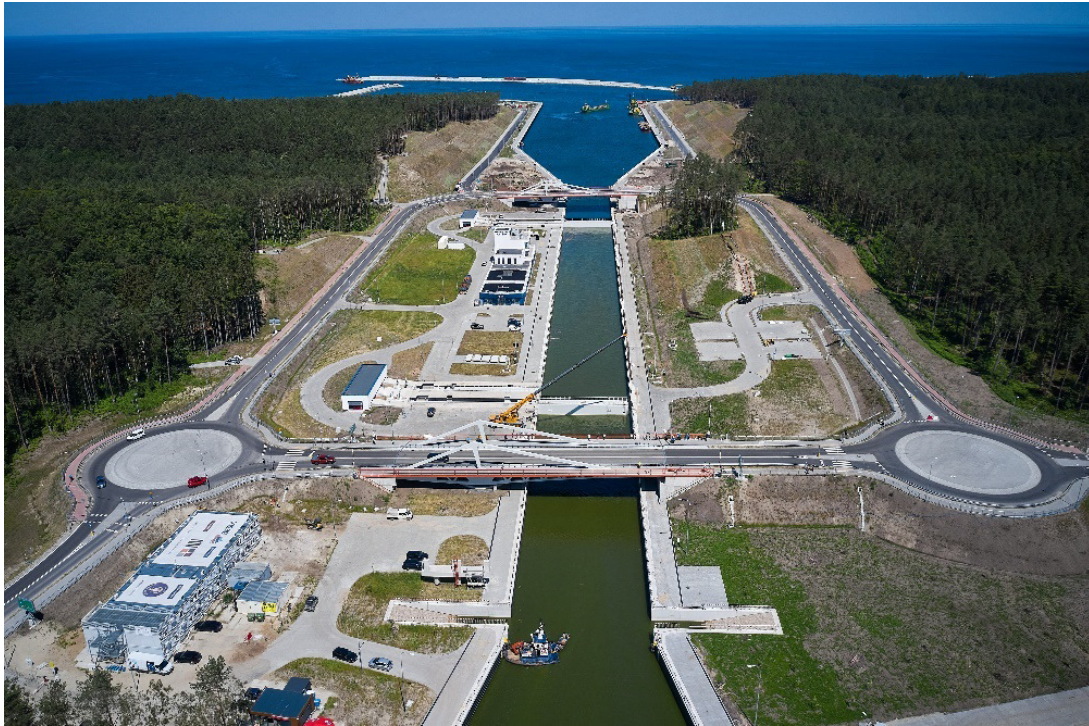
Figure 7. View of the completed canal through the Vistula Spit. Photo by EPA bought from Polish Press Agency.
