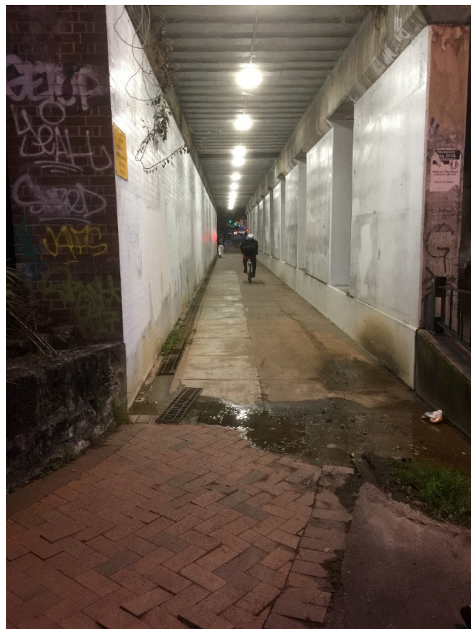
Figure 5. Underpass under the railway tracks in Upper Strathfield.
