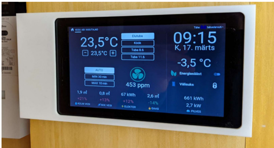
Figure 2. Smart home panel installed in the khrushchyovka-type apartments, 2021. Source: Courtesy of SmartEnCity project team.
