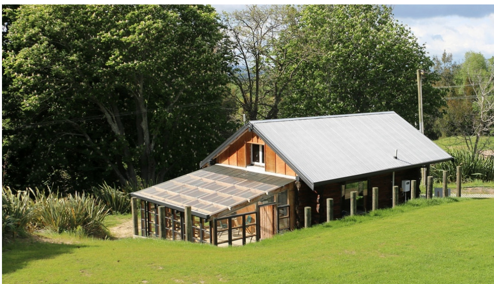
Figure 6. The LC after the renovation.
