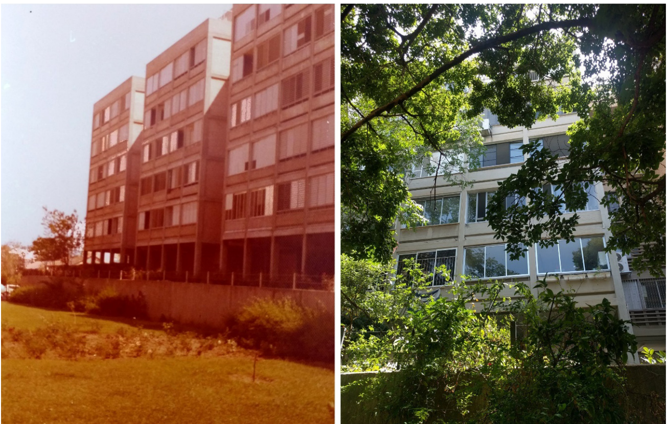
Figure 14. The central park, then and now. Left: Top row’s facade with original aluminium shutters on the balconies, 1970s. Right: Be’eri estate today, with vegetation hiding the top row’s facade. Source: Left photo courtesy of Nava Leibowitz.
