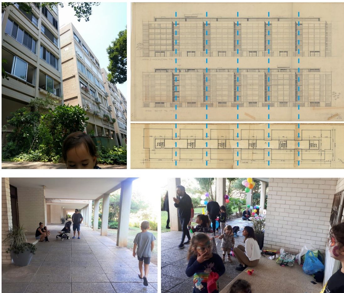
Figure 8. Facades and roof plan of one of the elongated buildings (40–50 Be'eri street). Note in the facades the recessed service balconies (dark grey) shaping the large building as a series of separate-looking volumes. Top: the facades' drawing, 1963; Bottom: roof plan, unknown year, with graphic additions by the authors. The building's design as a series of separate-looking volumes softens the large building's massiveness and produces a colonnade with extensive thresholds for each entry. Sources: A. Sharon (1963); photos by the authors.
