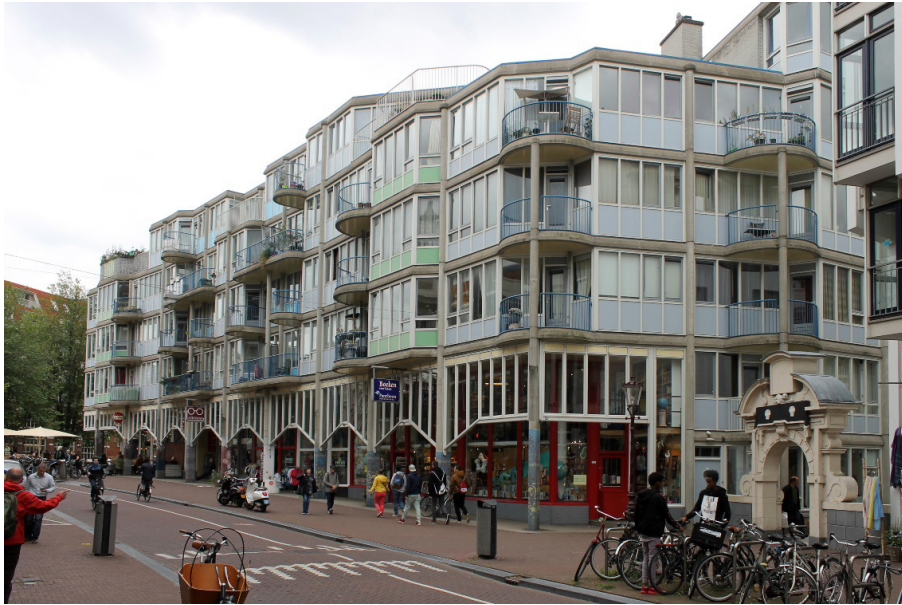
Figure 5. Sint-Antoniebreestraat (the Pentagon), 1969–1975, Amsterdam, by Van Eyck & Bosch. Source: Courtesy of Ronald Klip.
