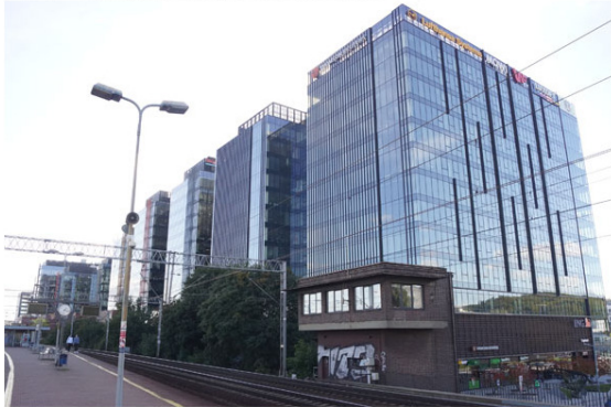
RAILTRACK AND STATION PASSING THROUGH
