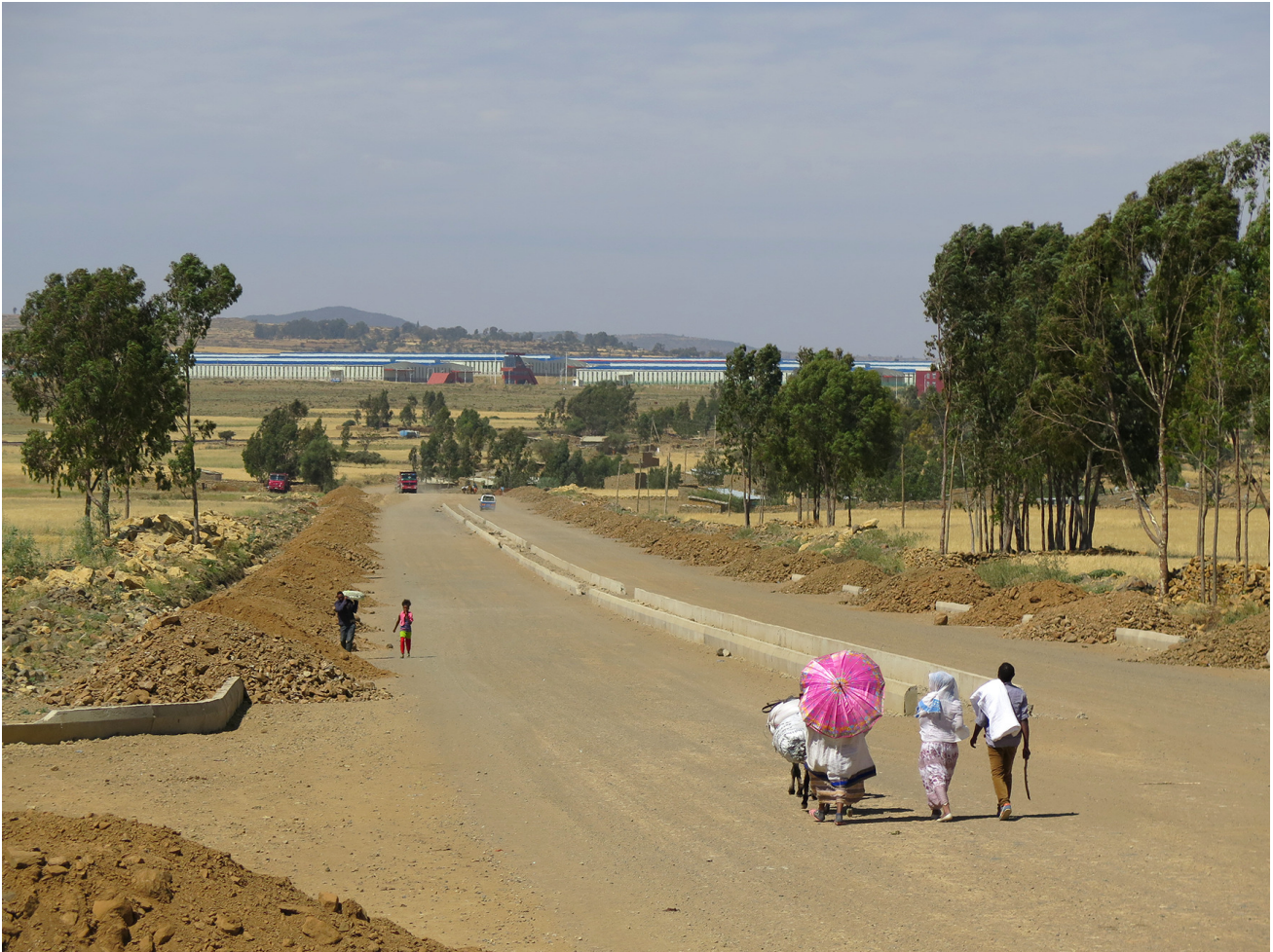
Figure 4. MIP and bypass under construction (2018).
