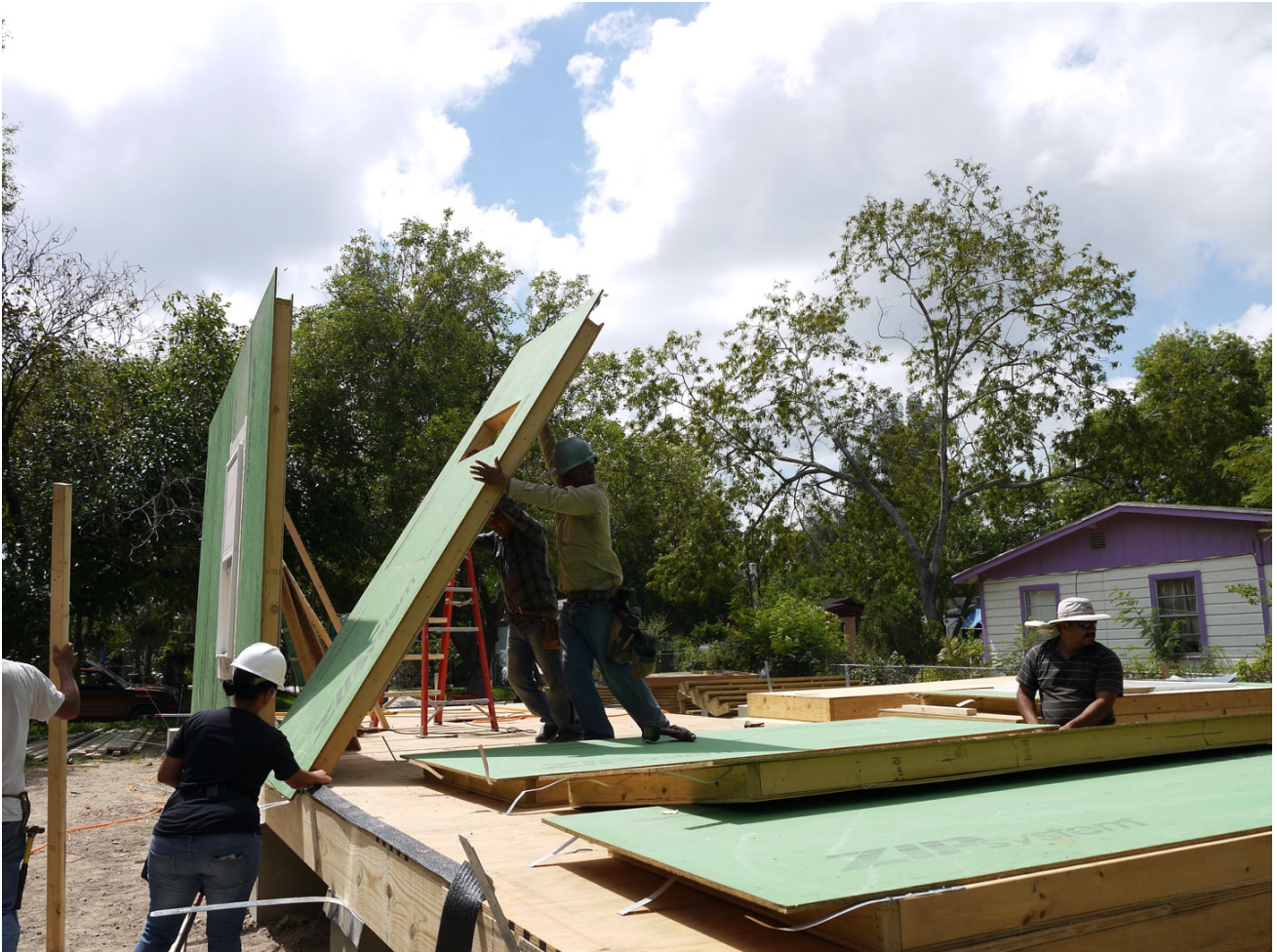
Figure 1. Photograph showing the installation of SIPs in the core of a RAPIDO prototype home. Source: bcWORKSHOP (2016).
