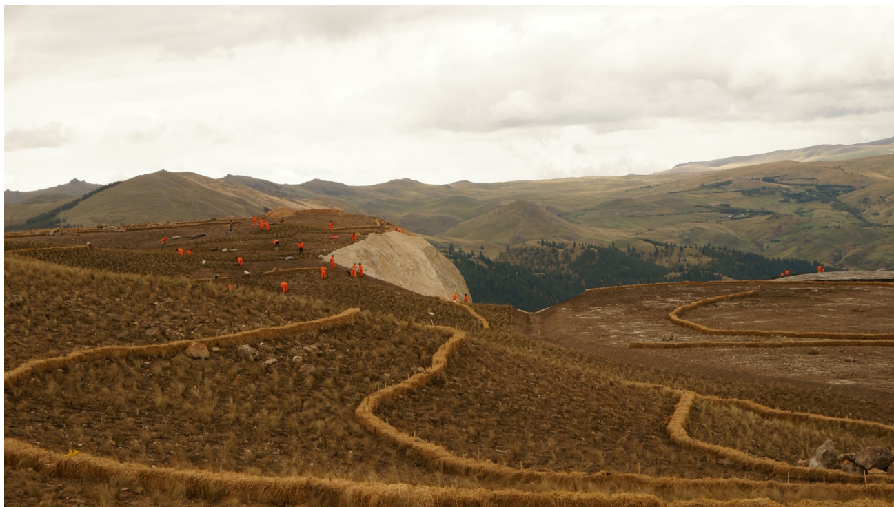
Figure 11. In 2015, excavated materials from La Quinoa pit served to re-contour its adjacent north rock waste piles while expanding operations south, towards the headwaters of the Grande River. The measures involved revegetation of the area with native pastures and mimicking the surrounding environment. Source: Photography by Margarita Macera.
