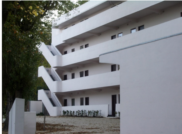
Figure 4. Wells Coates, Isokon Flats, Lawn Road, Hampstead, London, 1934. An application of the Existenzminimum idea in a lowrise collective housing block by a member of the MARS Group, with shared services. It housed Walter Gropius, Arthur Korn, and some other CIAM members in England in the mid-1930s. Source: Wikimedia Commons (2005).
