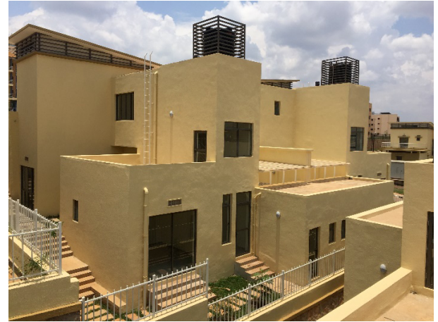
Figure 58. The Umudugudu Kigali Vision: Twin houses; back yard. Photograph by Manlio Michieletto.
