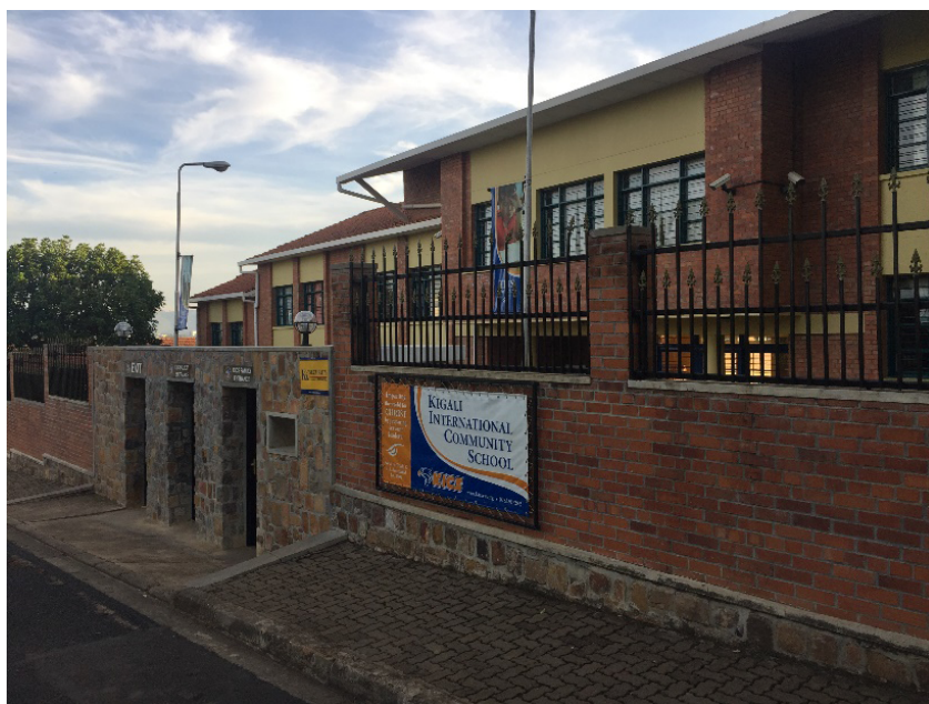
Figure 30. The Kigali 2020 International School. Photograph by Manlio Michieletto.
