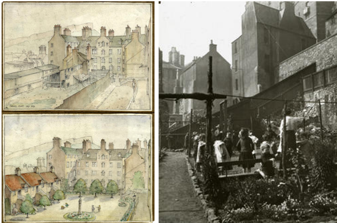
Figure 2. Repairs of Edinburgh Old Town Tenements, 1911. Photograph by Patrick Geddes and drawings by Nora Mears. Source: Patrick Geddes Papers (n.d.).
