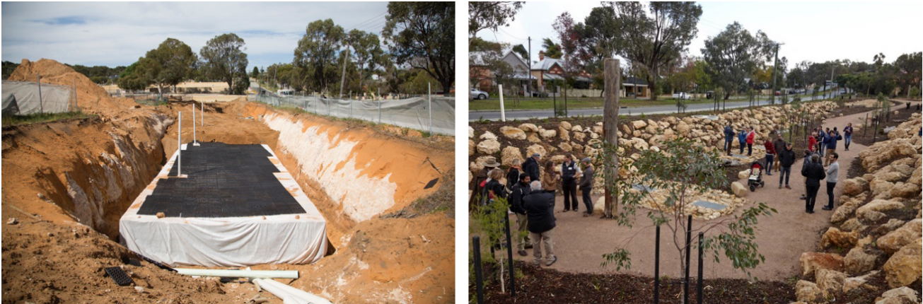
Figure 4. Left: installation of drainage cells as part of the retrofitting of the stormwater sump; right: the completed stormwater sump with a newly landscaped parklet for community use. Source: LandCorp (2015).
