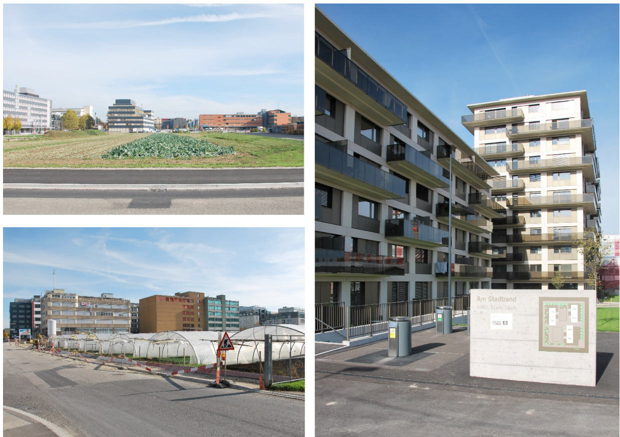
Figure 6. First building projects for the restructuring of the Hochbord area are already completed and represent high density housing projects. Source: author.
