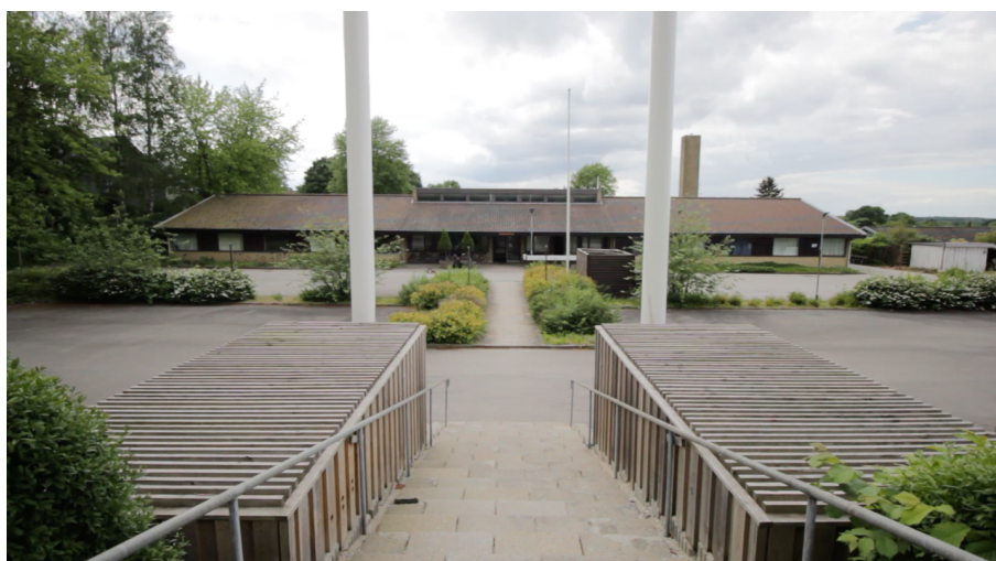
Figure 1. Former retirement home as seen from the street. May 2017.
