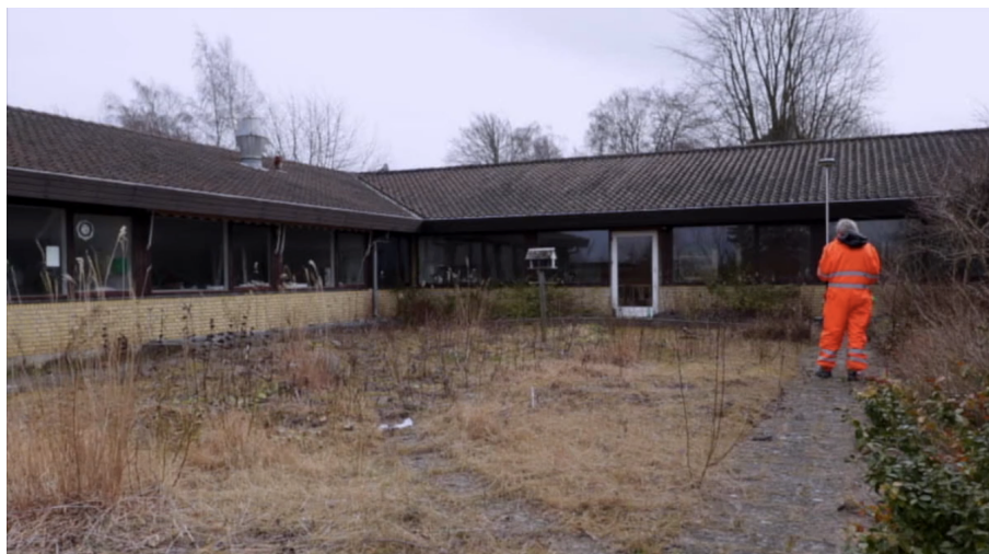
Figure 6. A surveyor measures the plot to prepare for the new construction project. March 2017.
