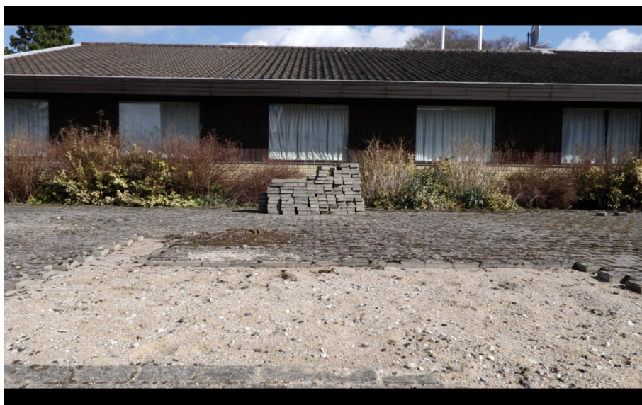
Figure 5. Bricks have been collected and stacked in the yard. March 2017.
