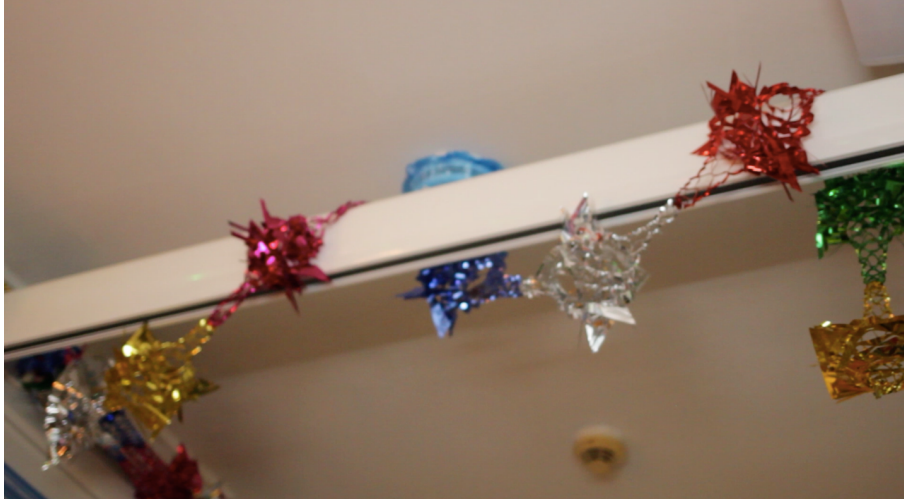
Figure 14. Decorations covering the hoist on the ceiling. April 2017.
