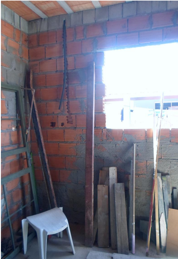
Figure 19. Case E, windows and high beams. Source: author's archive, 2013.
