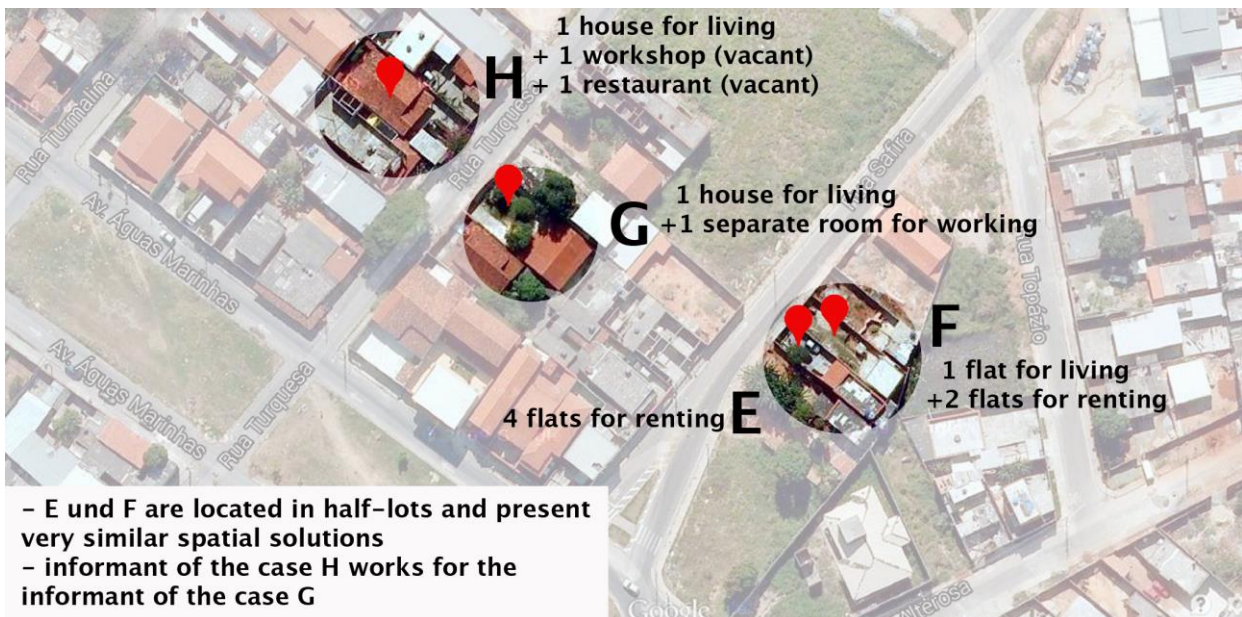
Figure 6. Cluster São Joaquim, Contagem. Buildings are unfinished, with some work or renovation still on course. Source: elaborated by the author, 2014.
