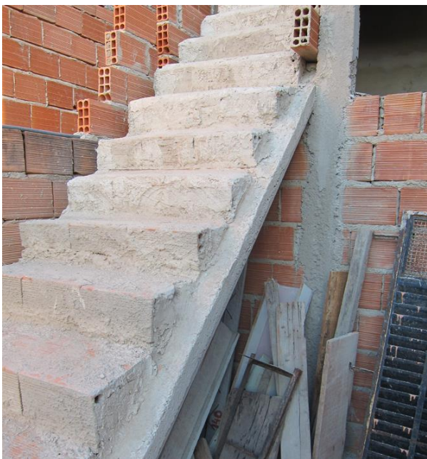
Figures 18a and 18b. Case E, building's stairs. Source: author's archive, 2013.
