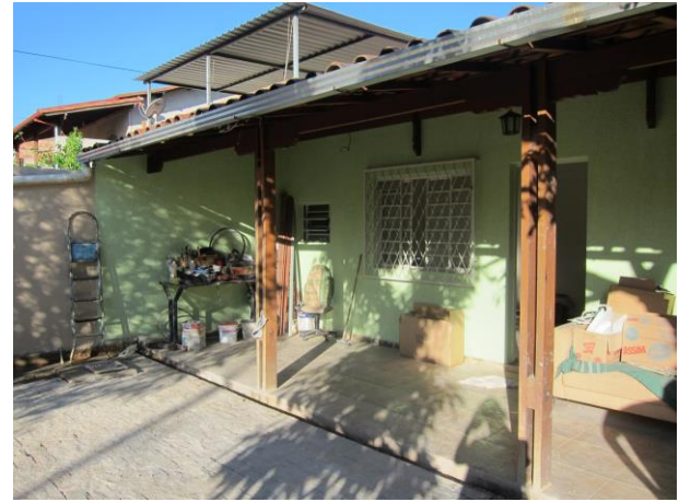
Figure 14. Case G, renovations in course, managed by the friend and neighbour, informant of the case H.
