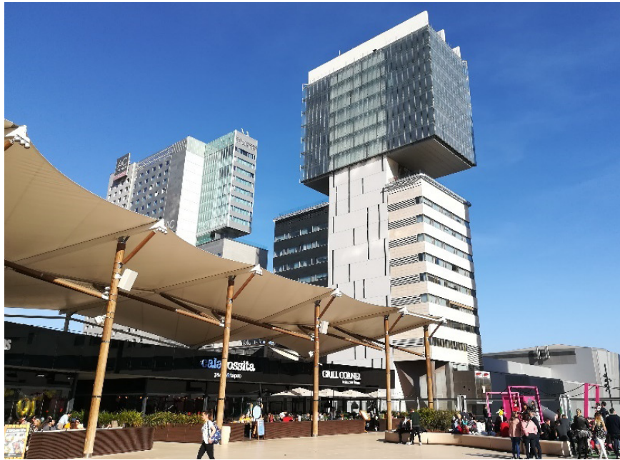
Figure 4. Shopping centre, hotel, and office block in Diagonal Mar (Barcelona).
