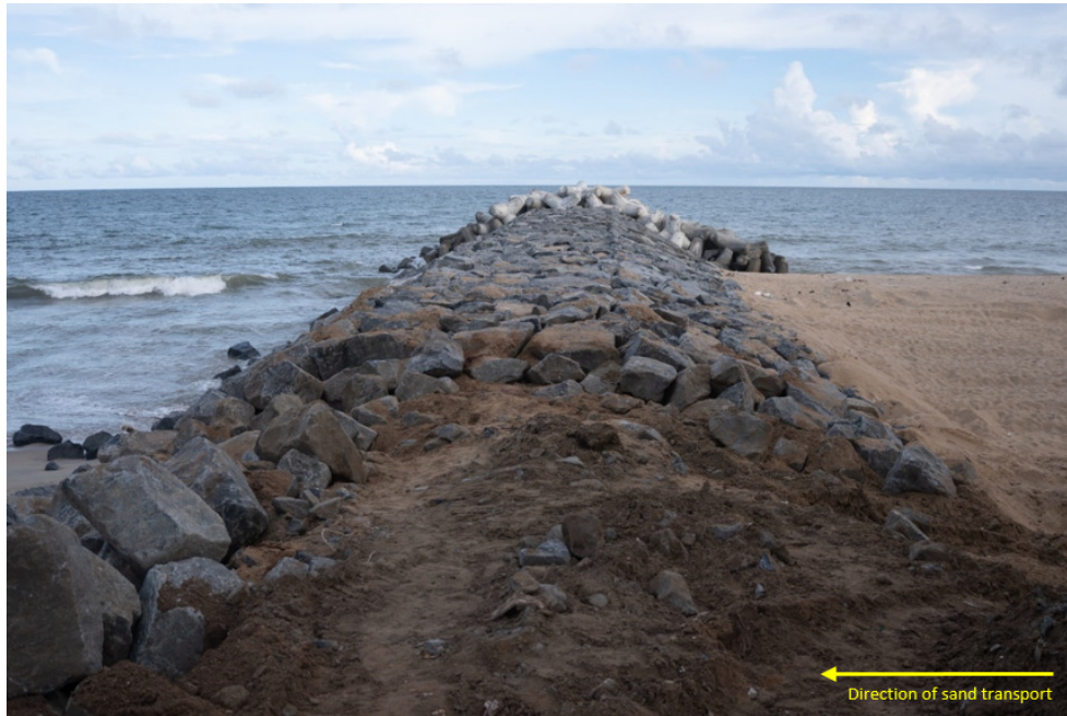
Figure 6. A groin in Bommayiarpalayam village is blocking sand movement northwards.
