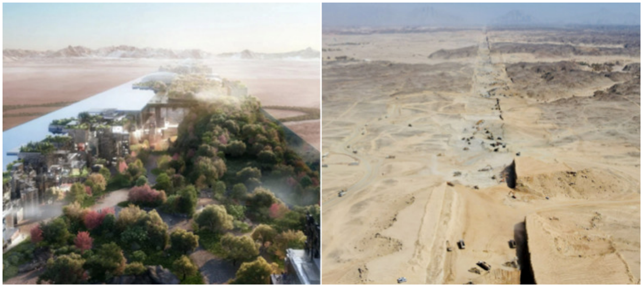
Figure 2. Contrasting The Line as a virtual experience and a physical construction. Both images are part of the promotional material publicly available on the development project and featured in the “progress” videos. Source: NEOM (2023a).
